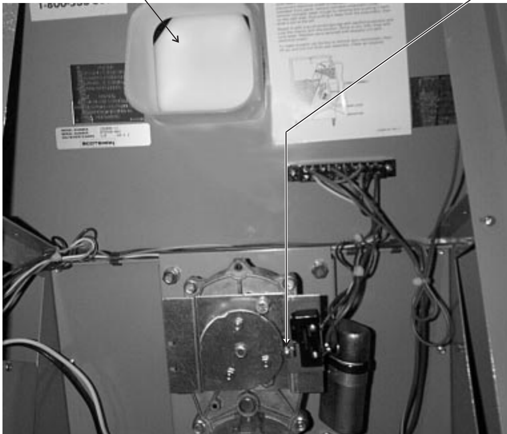
Correct Positions of Cam and Rotor at Rest
